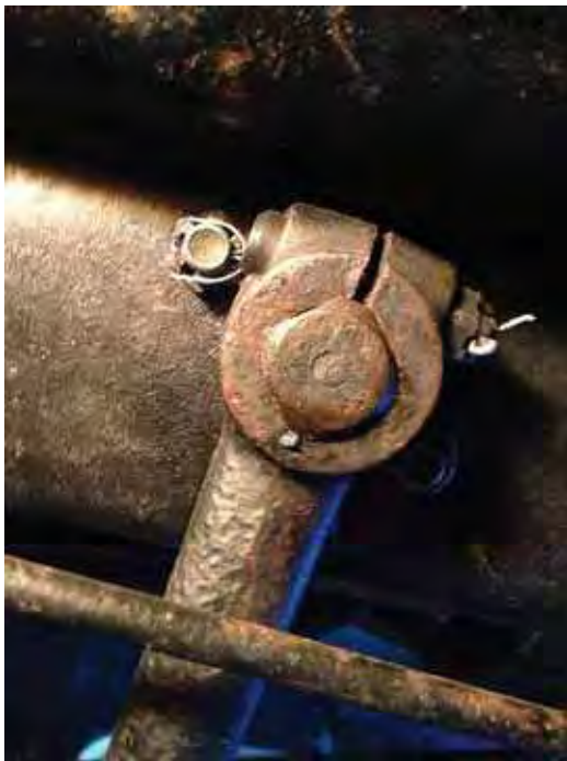
Remove cotter pin and castle nut from the pitman arm and remove it and then the two sector housing to frame castle nuts and bolts.
